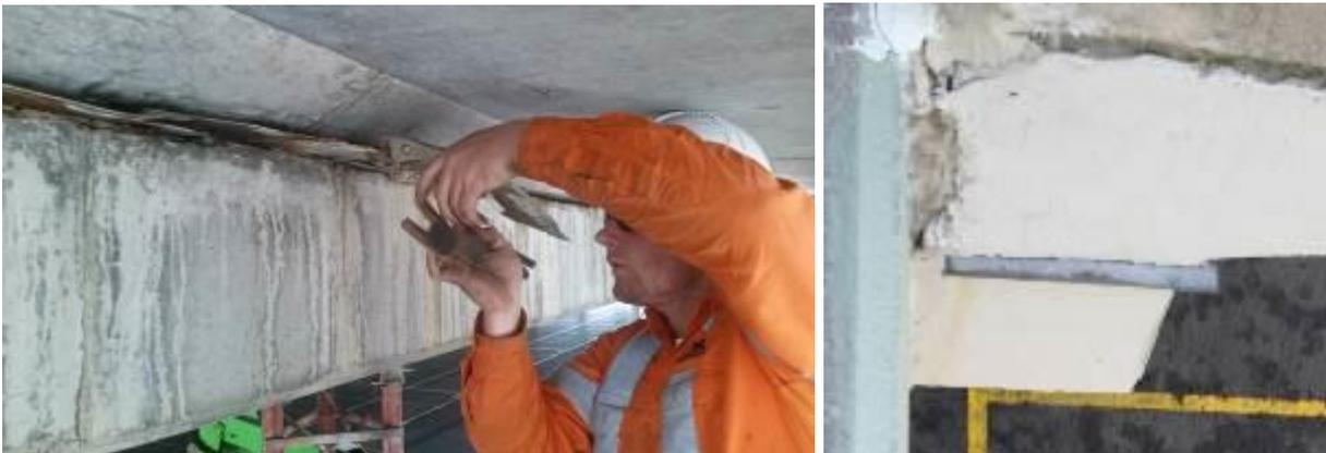
*Extraction of the old slip joint being removed by RKR Engineering team, left and close-up of the slip joint, right*
