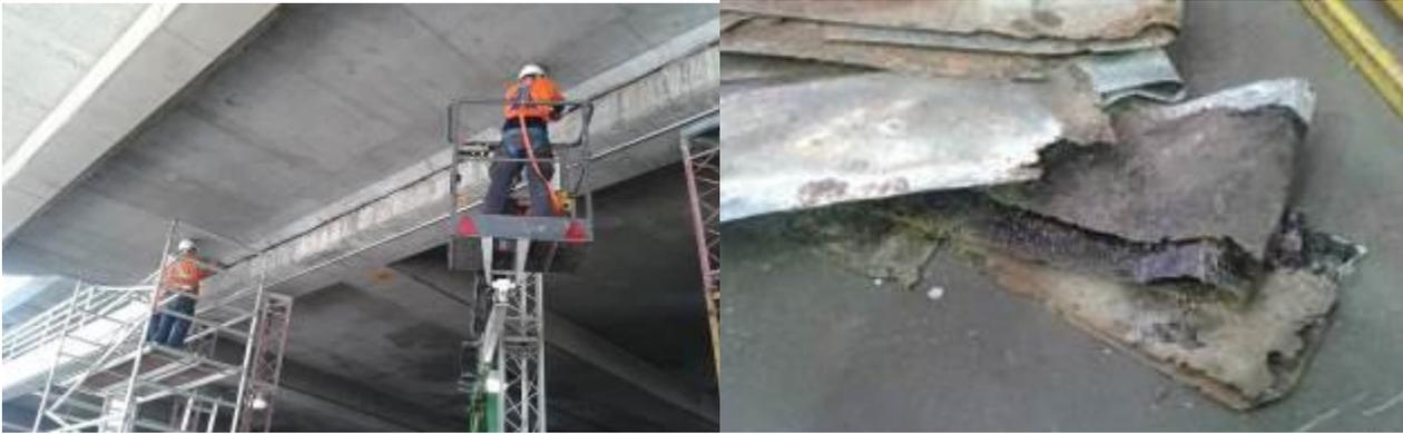
*Installing the new bearing, left, and the deteriorated original slip joint*
